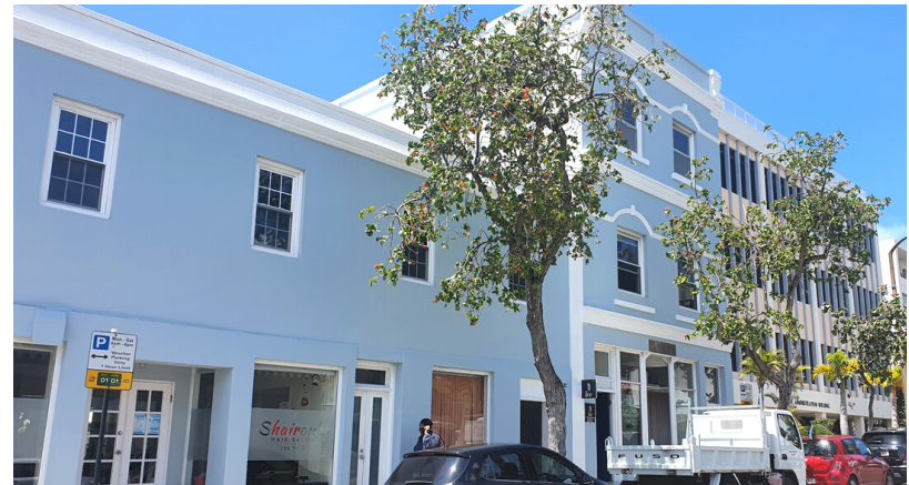
Hinson Hill Building, 34 Parliament Street
